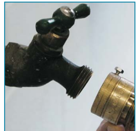
A hose bib without backflow protection can be easily protected with an anti-siphon adaptor.
